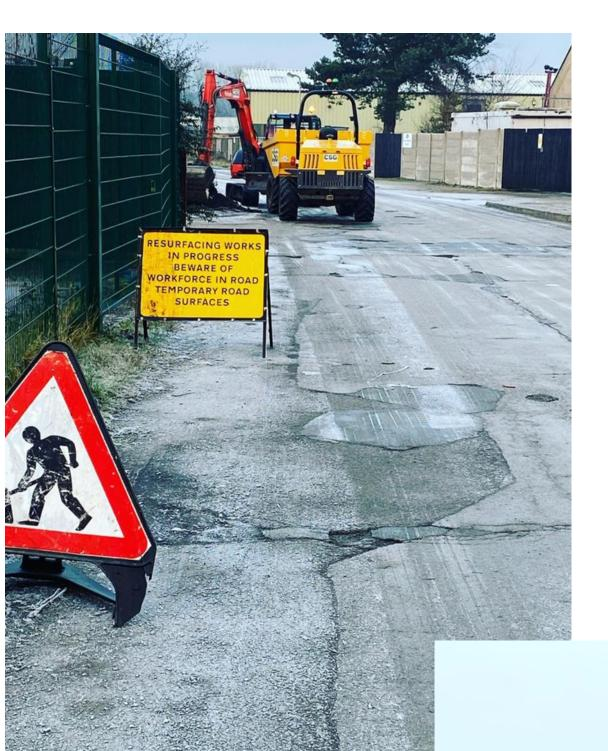
Our Work: Works included erection of traffic management, extensive verge clearance through reduced dig, road planing and removal of waste, resurfacing with binder and surface course, reinstating linemarkling. Improve the condition of roads for their heavy HGV traffic flow. Project completed within 36 hour timeframe with the road returned to service
