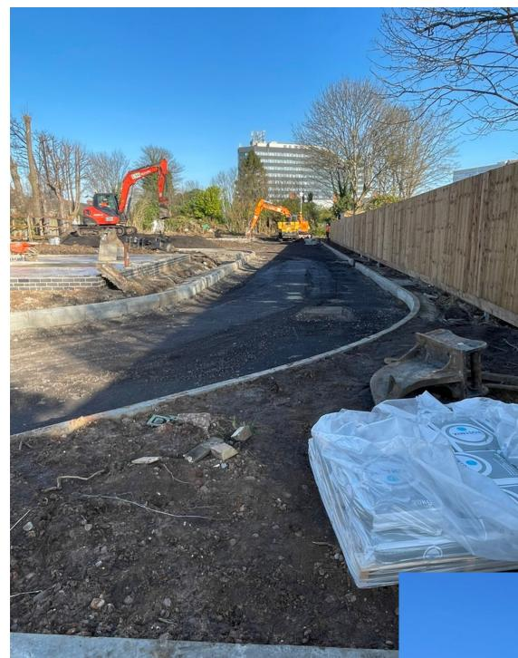
Our work: Enabling works including demolition and site clearance, Deep drainage, Attenuation and plot drainage, infrastructure including working with statutory undertakers to connect services Including electric, data and sewers through section 106 works. Foundations to DPC ready for modular build, Adoptable carriageway roads, car parks for each building.
