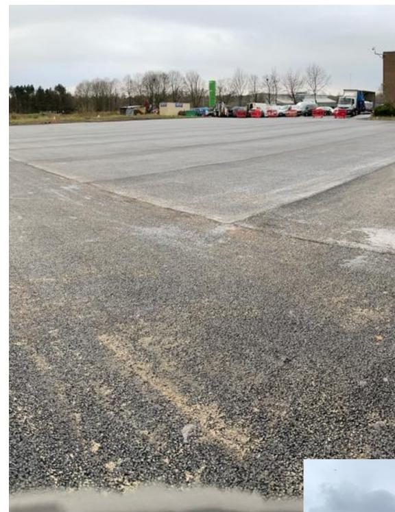
Our Work: Design and create new car park and roads around the building for tenants critically high HGV use, including site external drainage. Product used was Tarmac Ultiphalt HD.
